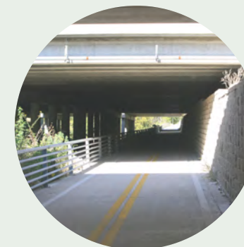
Terry Hershey Trail North high comfort crossing under I-10.
