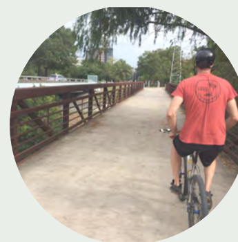
Terry Hershey Trail bridge over Buffalo Bayou.
